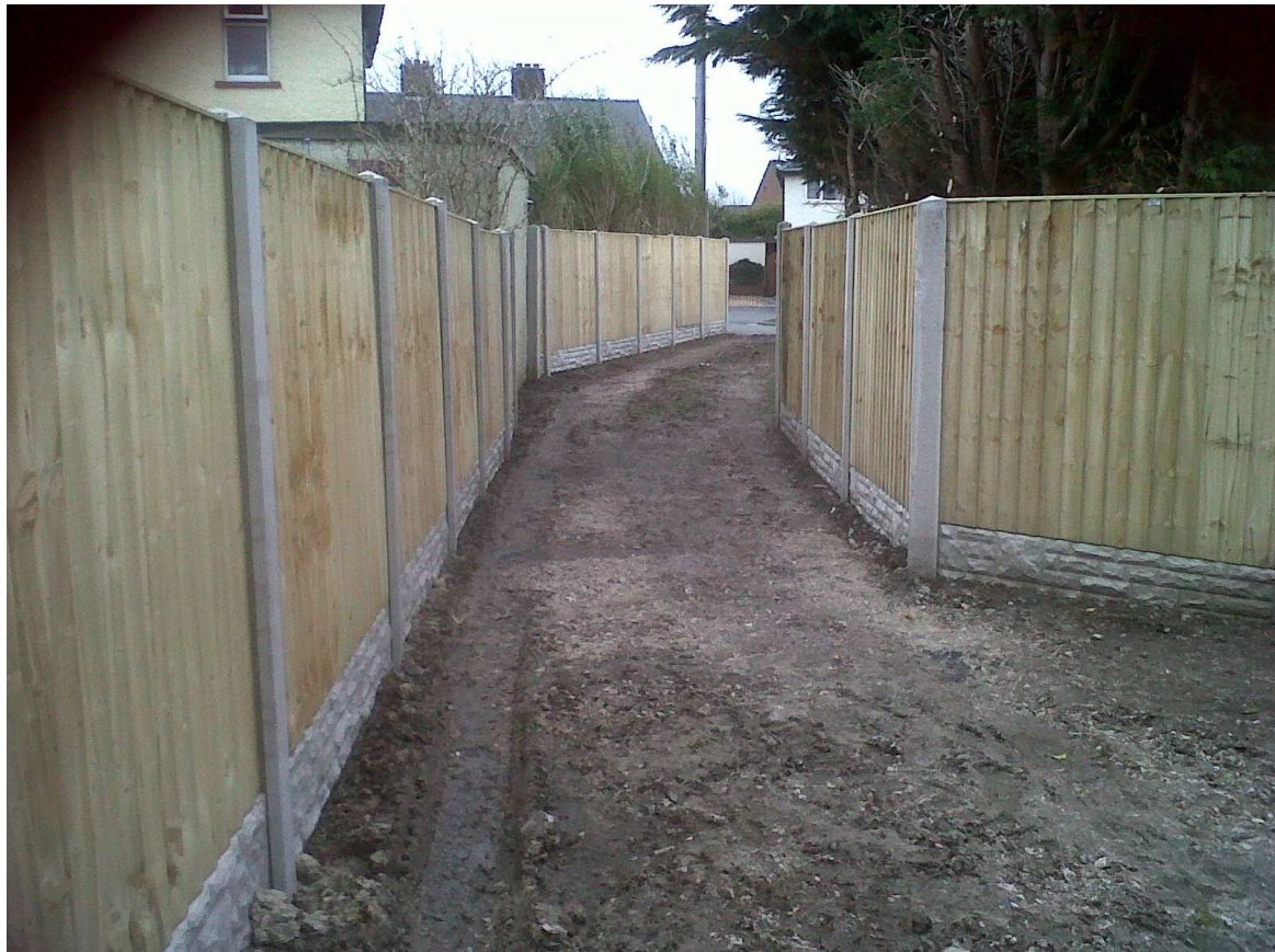
Beechwood road stage 2
