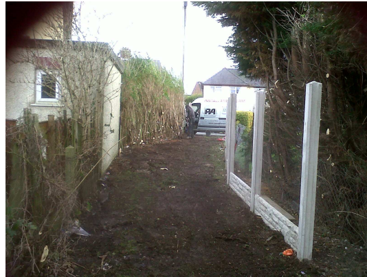
Beechwood road stage 2
